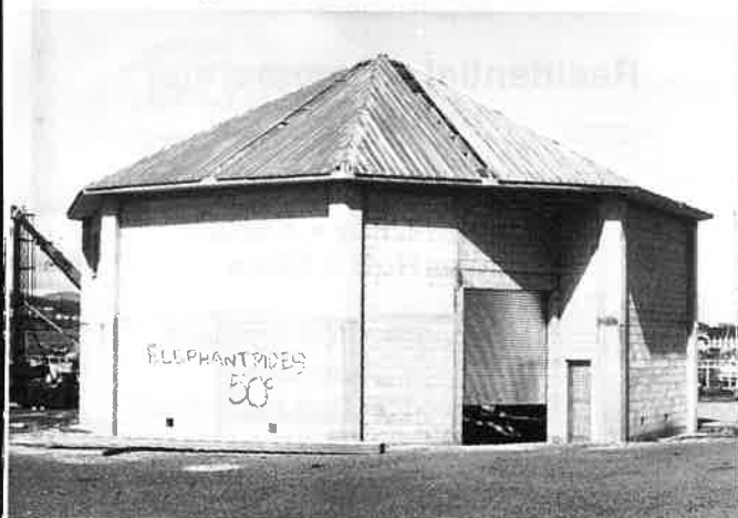
Wellington's innovative Sea Rescue Service Centre under construction at Evans Bay.
