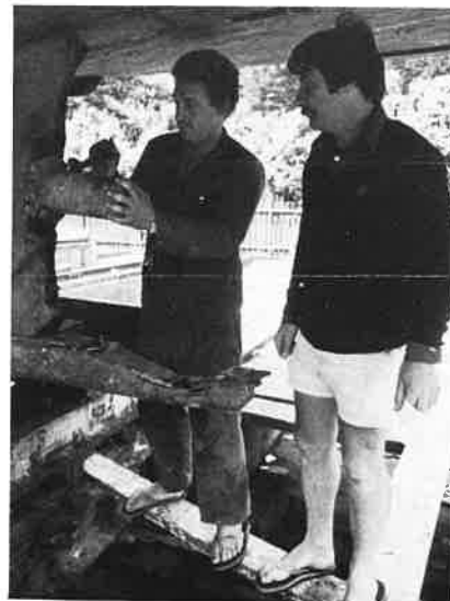
Grant Aikman (right) watches co-proprietor Phil Cox wield a spanner on a stern tube at the Shelly Bay Slipway.
